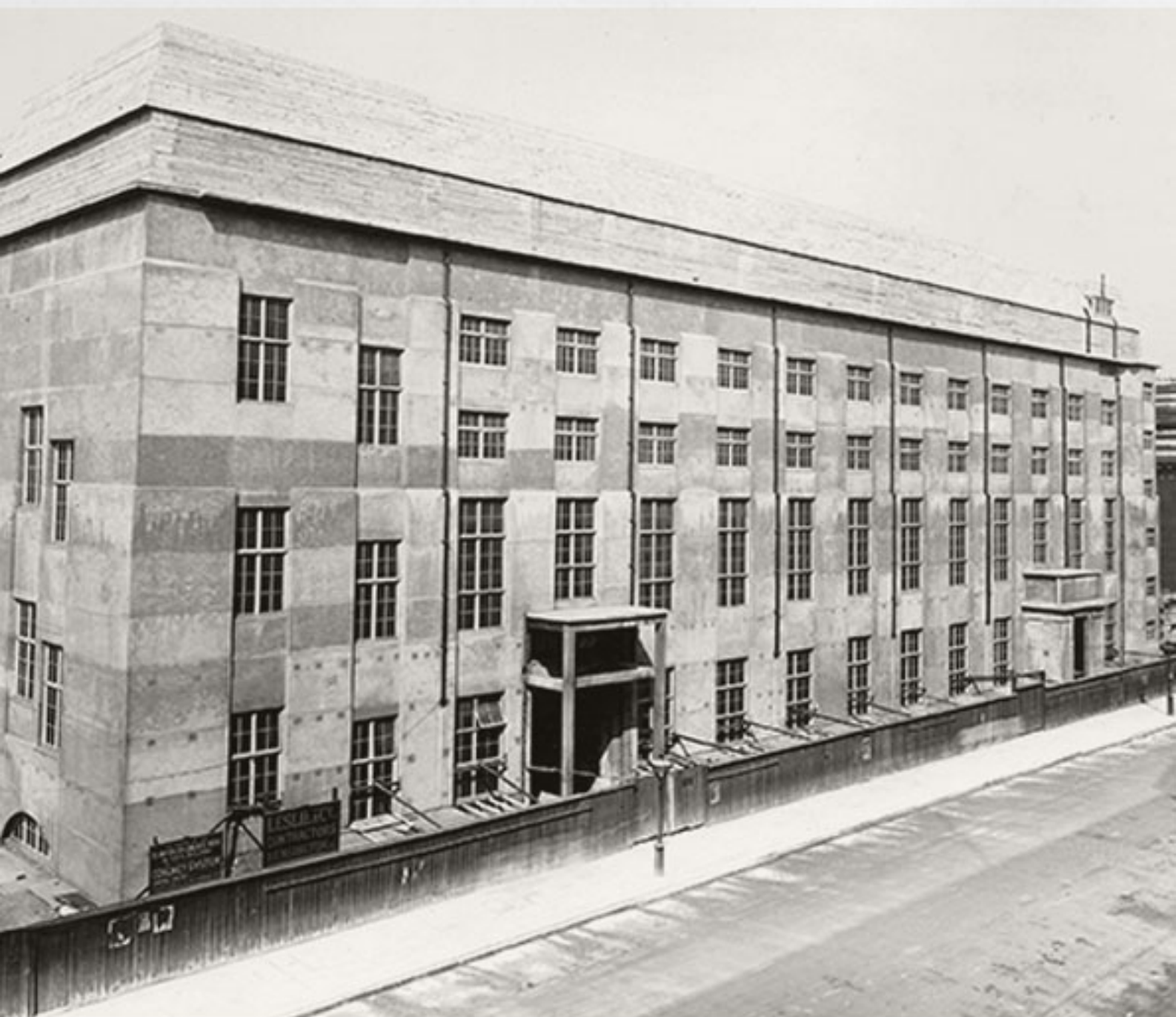
Construction of the East Block, Science Museum, London, 9 May 1919
